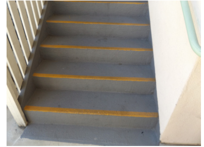
Typical Stair Condition
