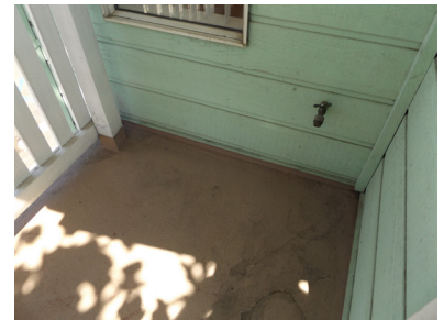
Typical Unit Balcony Surface Condition
