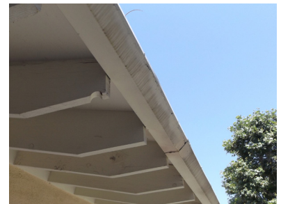
Gutter Condition, Typical
