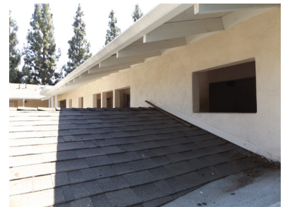
Typical Roof Condition
