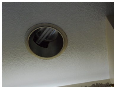
Typical Recessed Fixture
