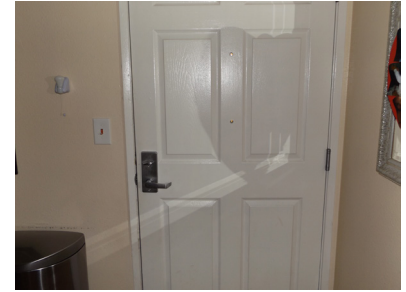
Unit Entry Door w/ Accessible Hardware
