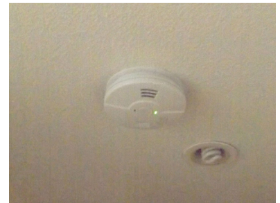
Typical Smoke Detector
