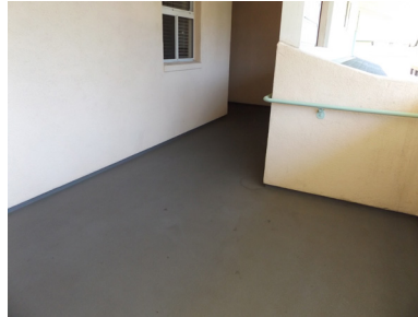
Typical Walkway Condition
