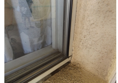
Track Condition, Typical
