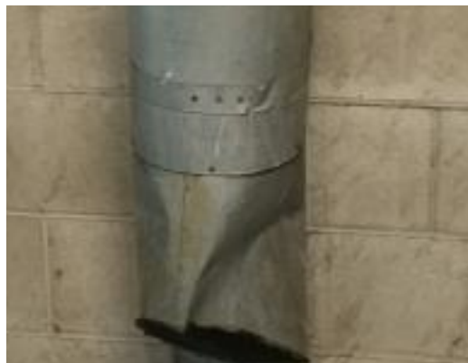
Damaged Ductwork
