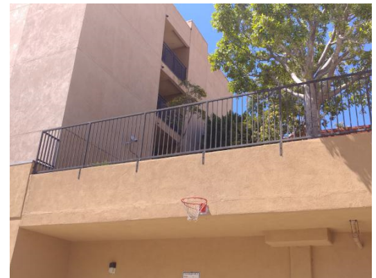
Fence Along Podium Level
