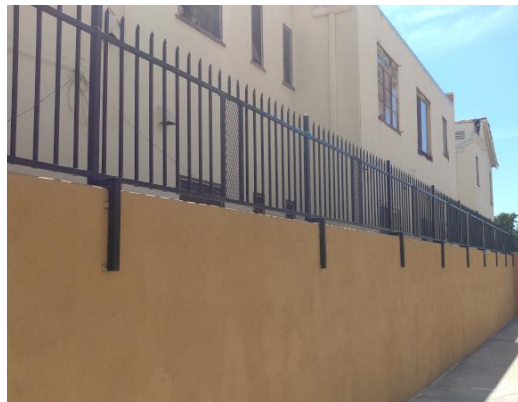
Iron Fence Topper on CMU Fence
